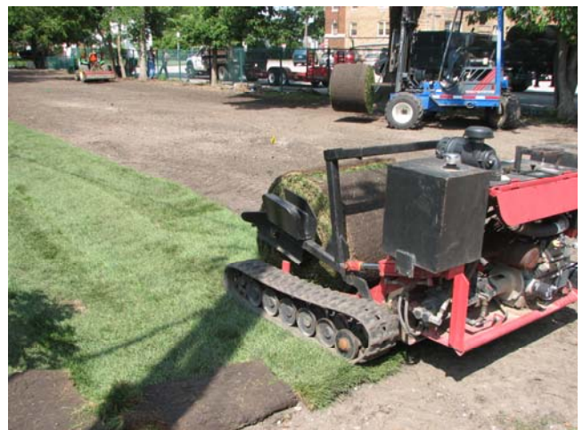
Laying the turf on Lindley Park
